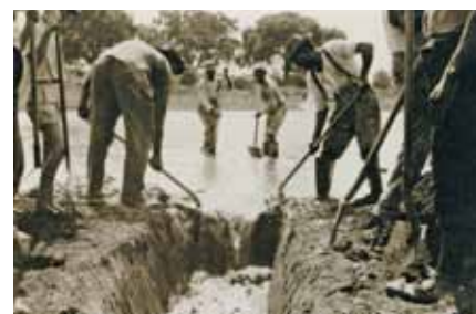
(Figure 9) Workers practising »vector control« by digging a drainage ditch (southern United States). Source: CDC (1920s)
